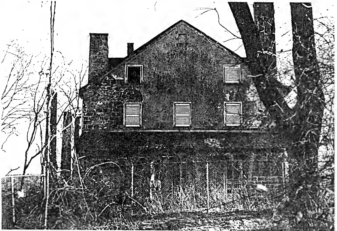
Figure 12: North Elevation of the Pawling/Wetherill House, 1995.
